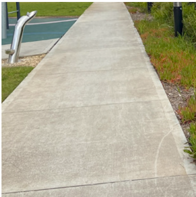
Concrete footpath- Broom finish to match existing
