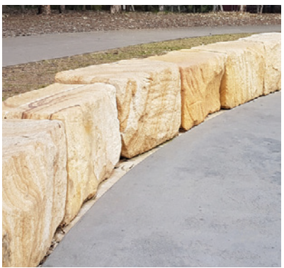
Sandstone dimension block wall
